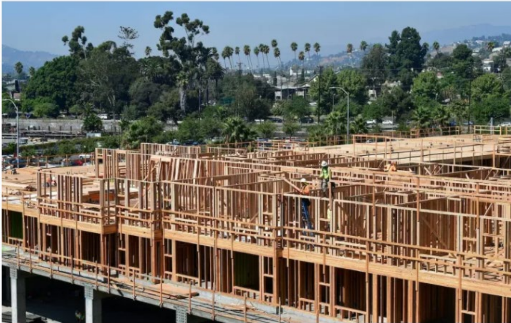
CONSTRUCTION WORKERS BUILD A MULTIFAMILY IN LOS ANGELES IN 2019.
