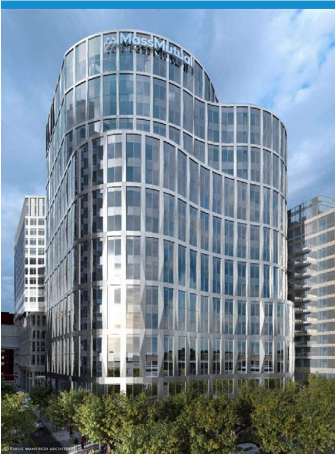
The new MassMutual Boston building features a striking curvilinear façade with faceted panels that facilitate enhanced thermal performance of the building envelope, accentuate the building's curvature, and capture the shifting reflections of sunlight and shadow. Rendering © Elkus Manfredi Architects
