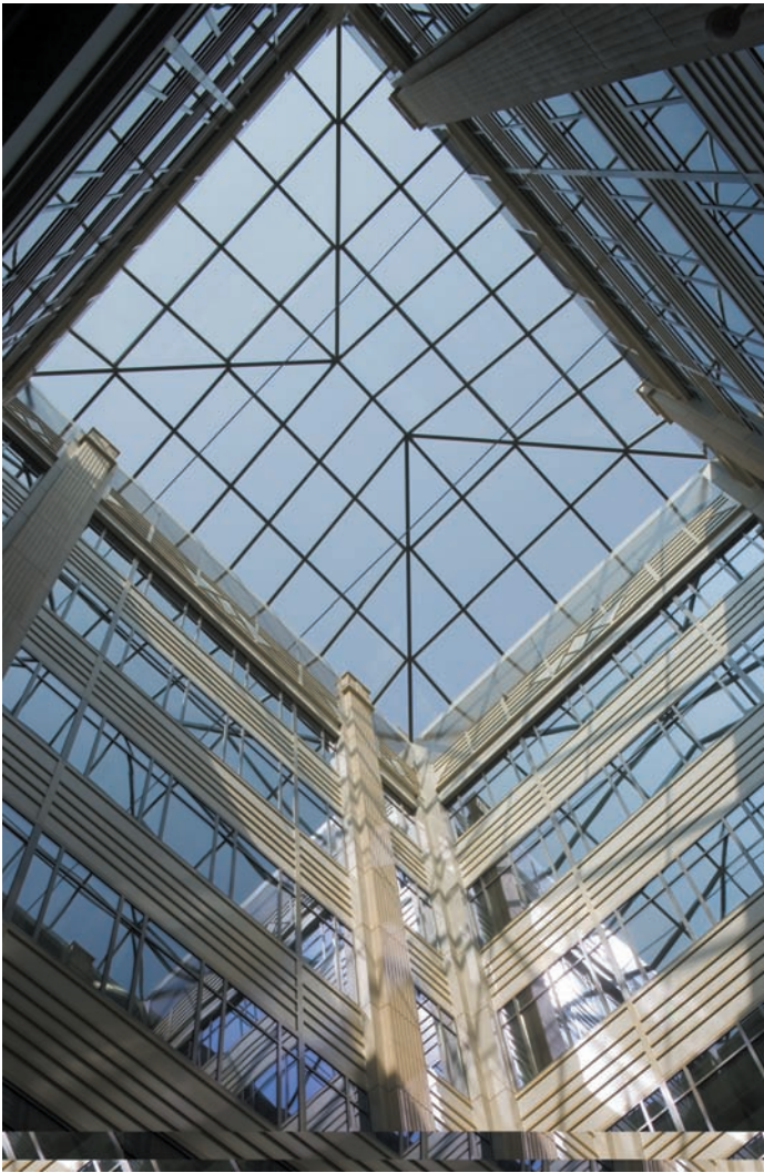
A new approximately 36x40-ft. skylight tops the lightwell in the center of the galleria, bringing natural daylight into the building.
