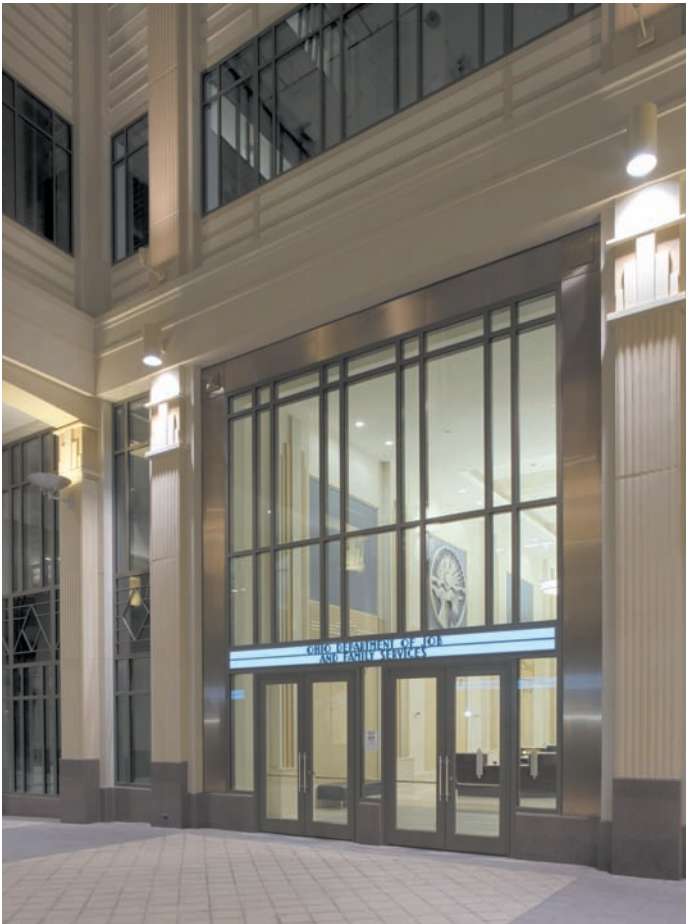
The entrance to the Ohio Department of Job and Family Services is located in the gallery under the lightwell.
