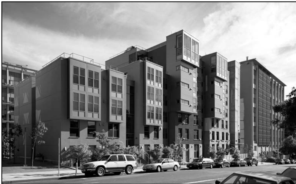
Infill buildings contribute to a pedestrian-friendly streetscape. Photo courtesy of Peter Aaron/Esto and EHDD Architecture
